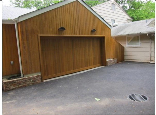
Backyard dry well showing driveway runoff also as a source.
