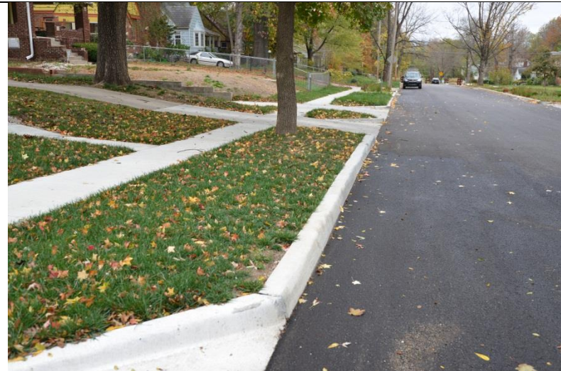
Upgradient from rain garden
