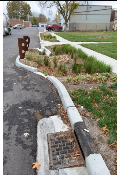
Towards cascade from next downgradient rain garden and drain inlet
